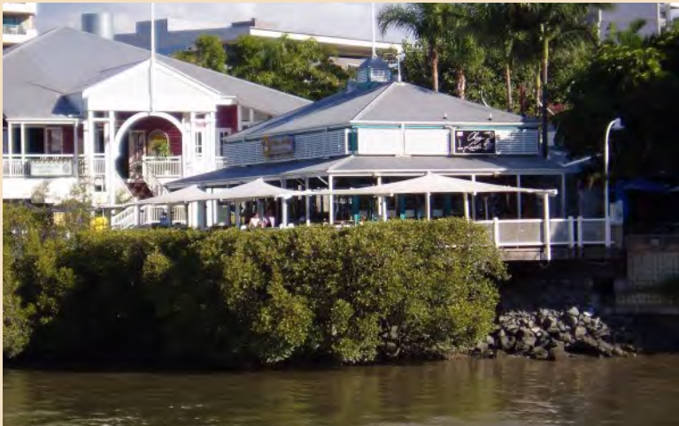
Mangroves along your seawall or rip rap provide additional fortification to the cement and rock structures.
